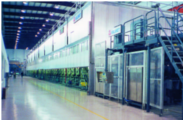
The new PM5 at Nanping Paper Mill
